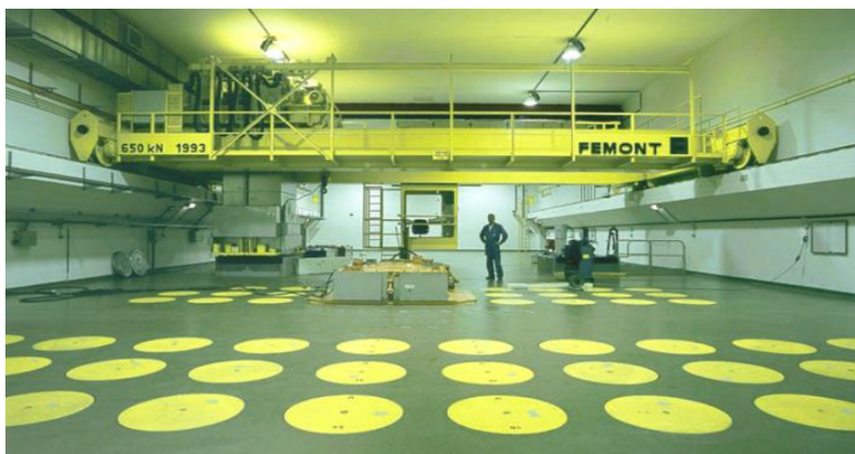
Storage of HLW, Belgium, (courtesy of BELGOPROCESS)
